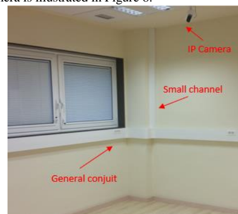
FIGURE 8. A corner of the Smart Lab with the central conduit and the small channel to the roof
